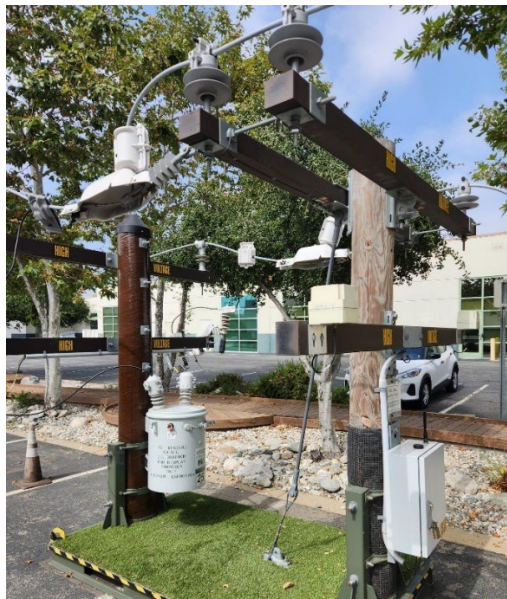
Electric distribution poles which have wildfire protections
